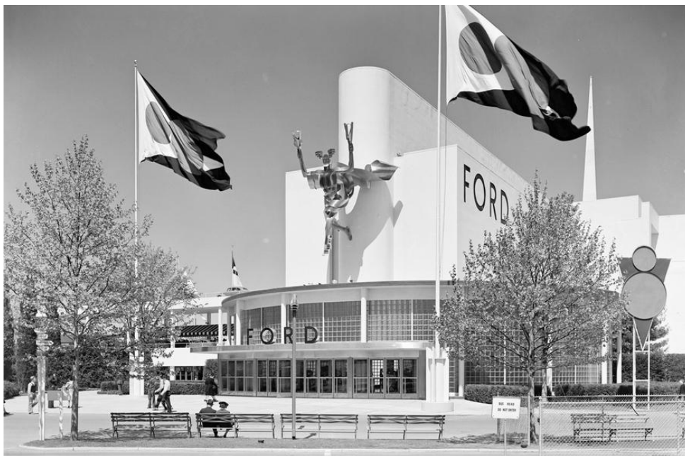
Ford Motor Building entrance, May 12, 1939. #
