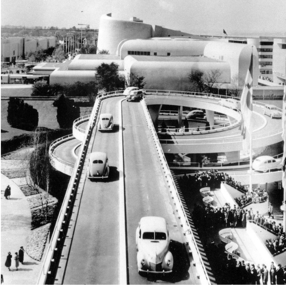
"The Road of Tomorrow," an elevated highway of cork and rubber composition, at the Ford Exhibit at New York's World Fair in 1939. #
